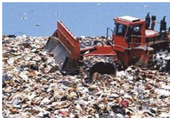
Very Top Of Above Landfill Showing Waste Spreading And Compaction Activities
