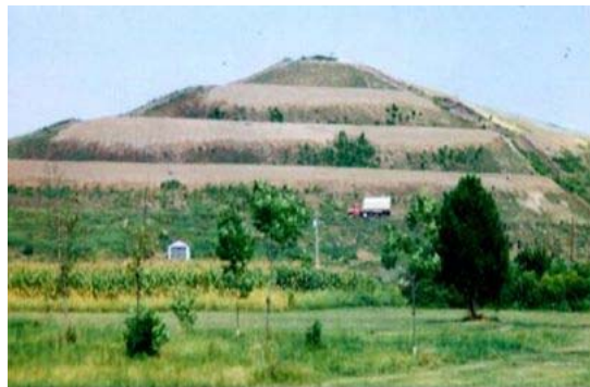
Typical Active Landfill Nearing Its Fill Capacity
