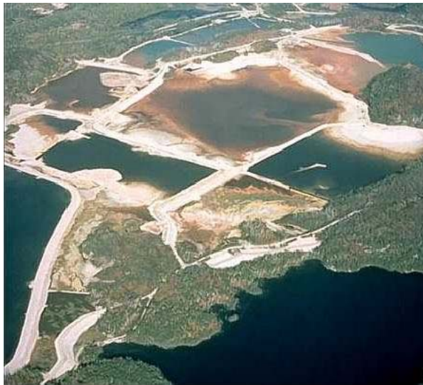
Typical Tailings Ponds
